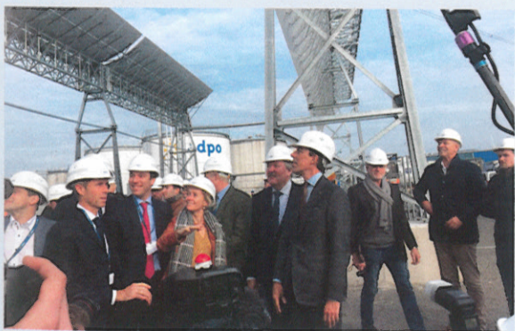
The Port of Antwerp inaugurated on October 23, the first solar concentrator farm in the European process industry, generating eco-friendly heat from concentrated sunlight that can be used by industrial companies.
